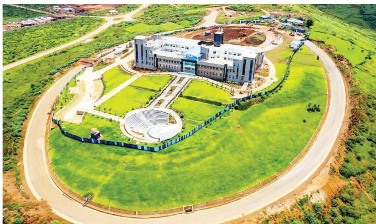
Construction work going on at Kigali Innovation City
