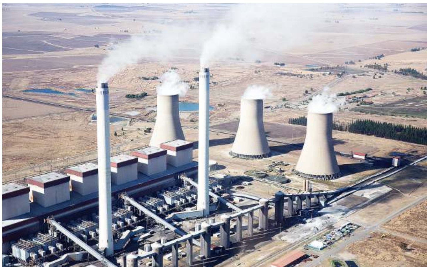
Eskom's coal fired power plant in Johannesburg.
