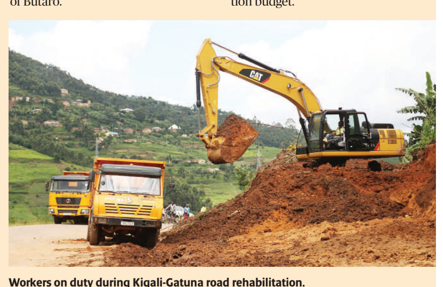
Workers on duty during Kigali-Gatuna road rehabilitation.
