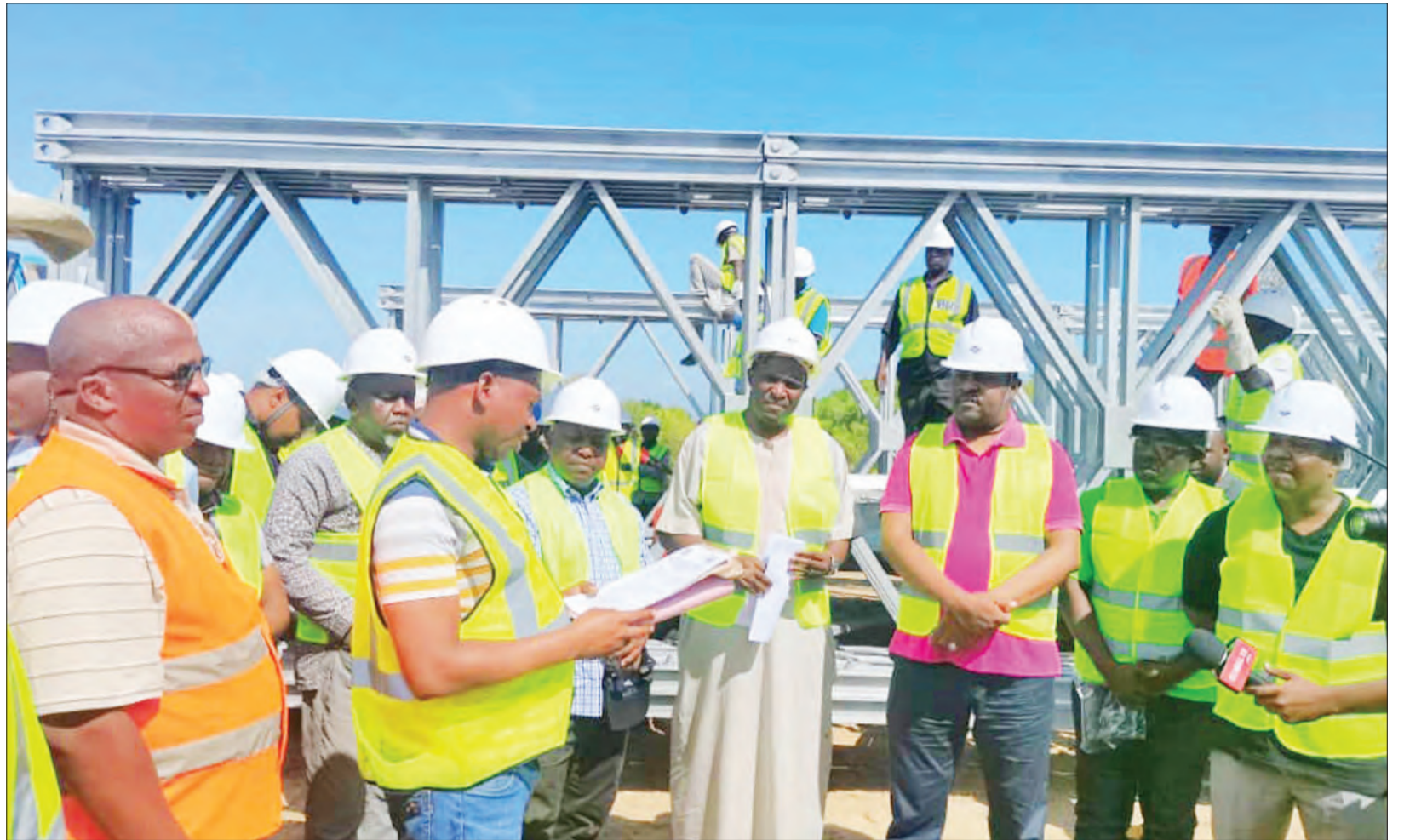
Engineer Leopold Runji (6th-R) briefs Coast regional commissioner Abubakar Kunenge (3rd-R) yesterday on progress on the construction of Mbuchi bridge in Kibiti District. Photo: Correspondent Julieth Mkireri
