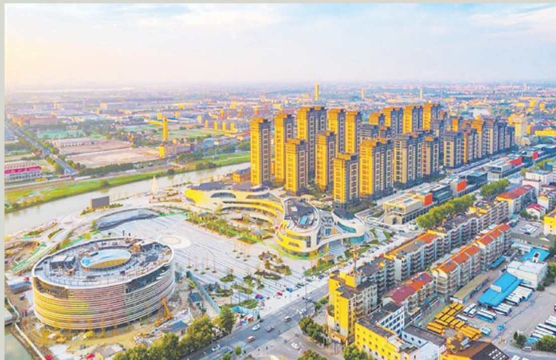
Photo taken in July 2021 shows Ditang community in Nanxun district, Huzhou, east China's Zhejiang province after low-carbon renovation. File photo very beginning of construction.
