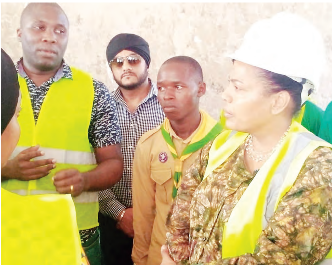
Dar es Salaam City Council engineer Isalia Edmund (L) briefs Angelliah Kairuki (R), Minister of State in the President's Office (Regional Administration and Local Governments), yesterday on ongoing construction work at Liwiti Secondary School. Photo: Guardian Correspondent
