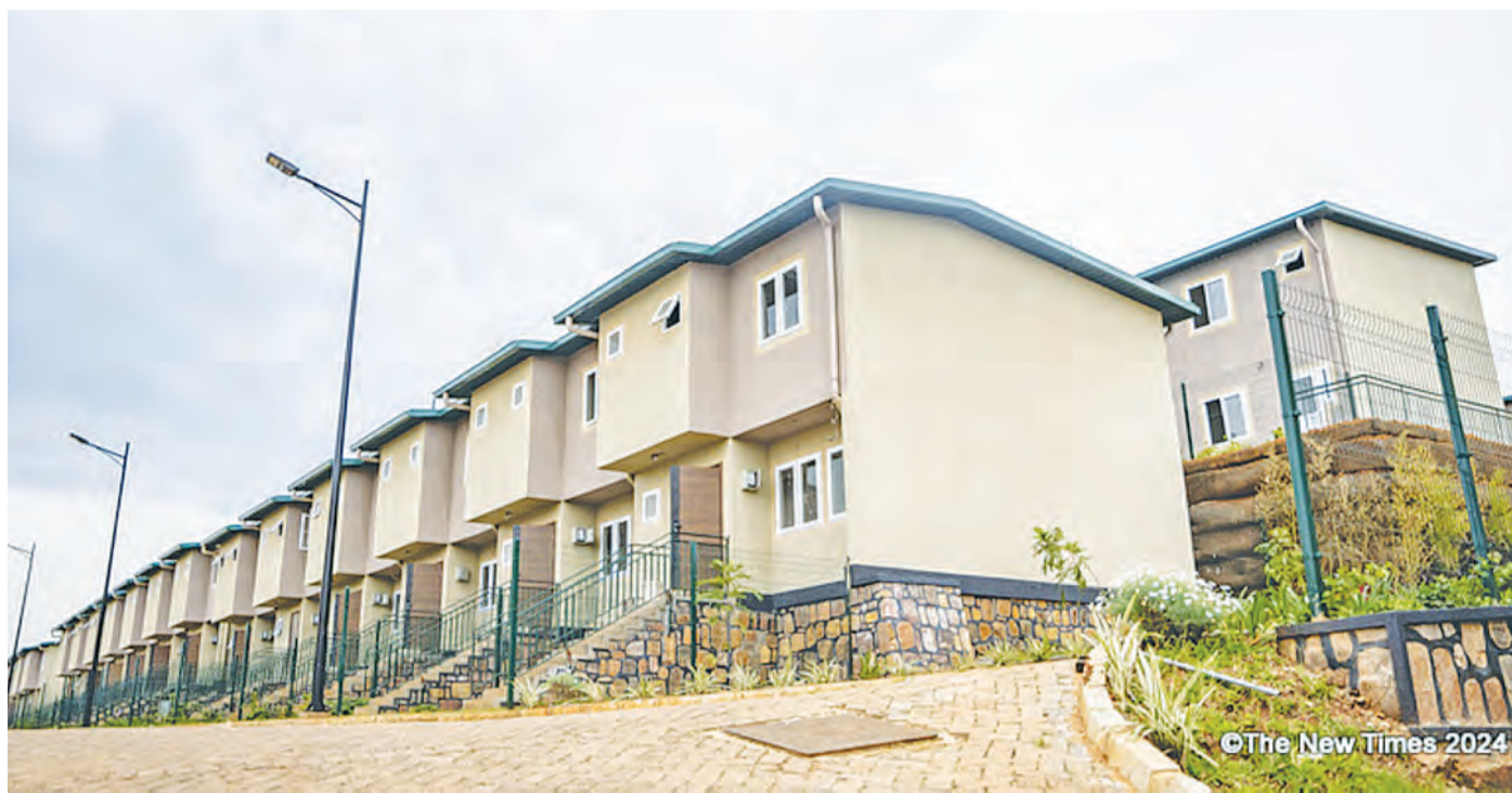
Tens of housing units at Bwiza Riverside Homes in Karama, Nyarugenge District.
