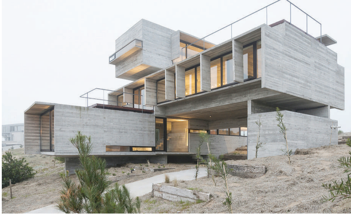
A concrete structure. Photo: Daniel Mac Adden
