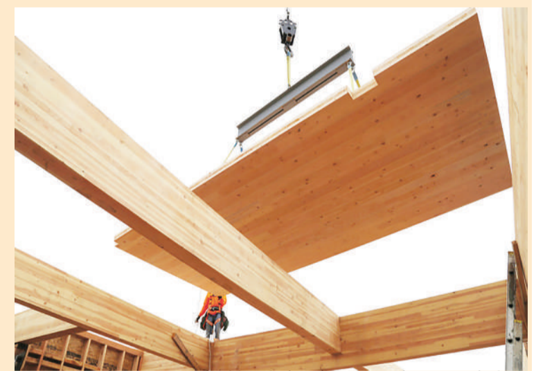
In the search for more sustainable solutions in construction, mass timber continues to take hold. Photo: Courtesy of LEVER Architecture
