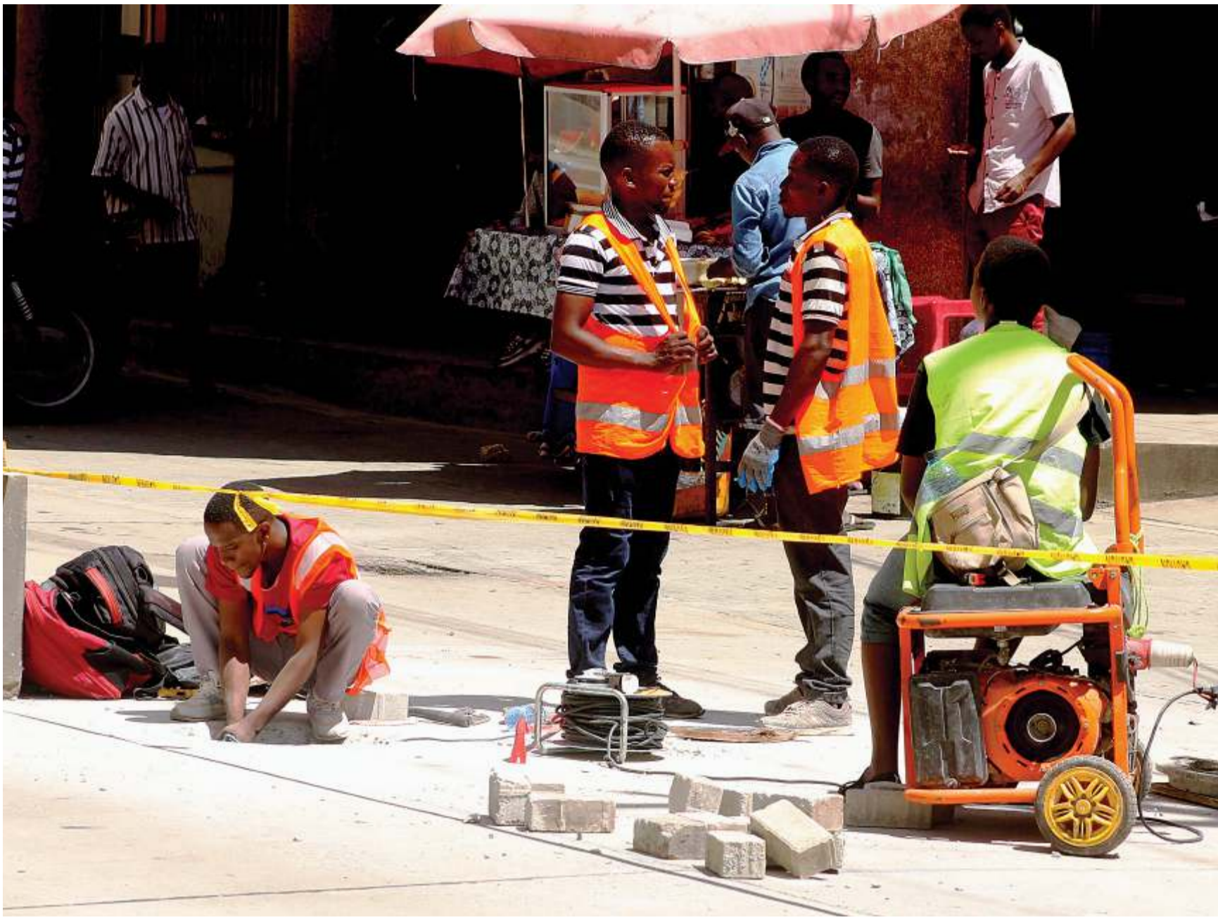
Dar es Salaam rapid transport bus project workers rehabilitate a sewage system in downtown Kisumu area yesterday. Photo: Correspondent Jumanne Juma
