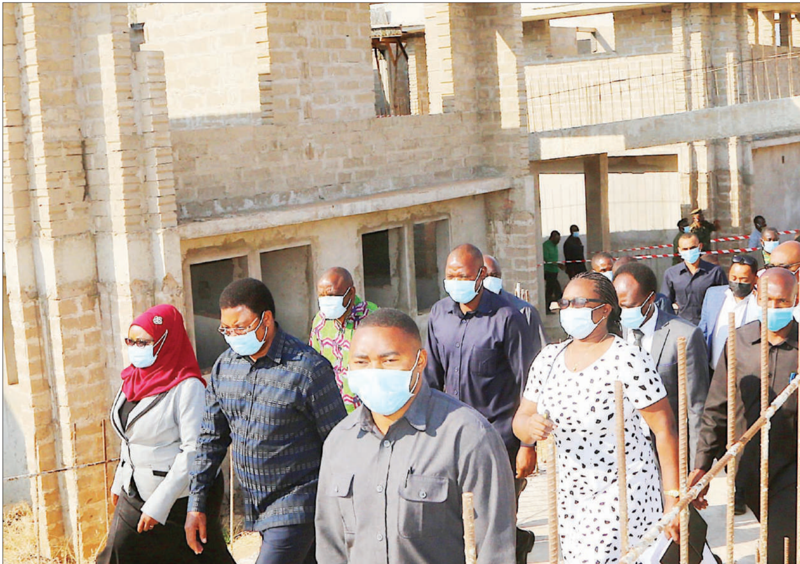
Prime Minister Kassim Majaliwa inspects the ongoing construction of Katavi Regional Referral Hospital at Rungwa in Mpanda district yesterday. Left is Katavi Regional Commissioner Mwananvua Mrindoko. Photo: PMO
