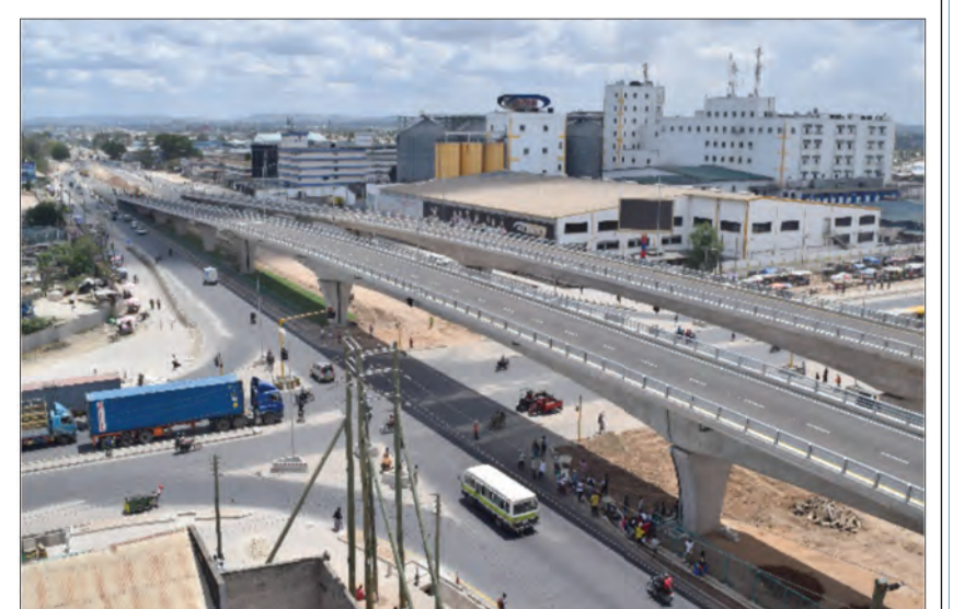
Mfugale Flyover (Source: JICA)
