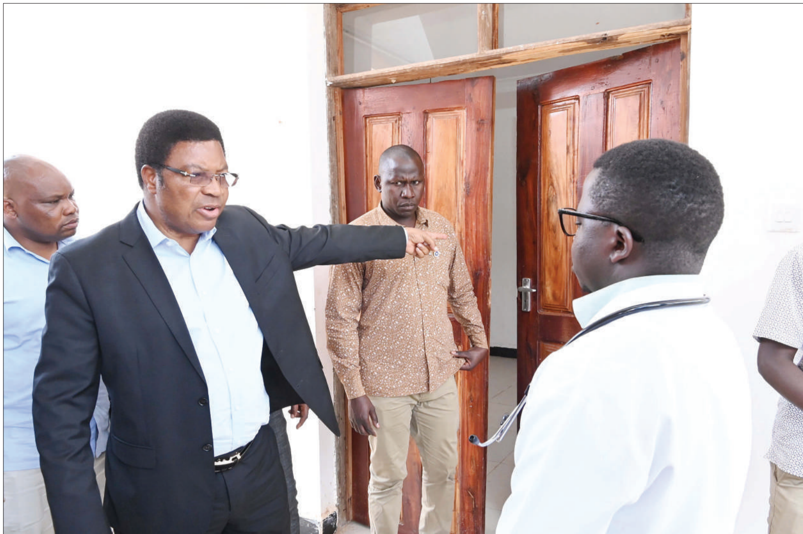
Prime Minister Kassim Majaliwa visibly far from impressed upon seeing a faulty door to the operating room at Namtumbo District hospital in Ruvuma Region yesterday, demanding an rectification of the situation. Right is the hospital's medical officer, Dr Christopher Wabwarumi. Photo: PMO
