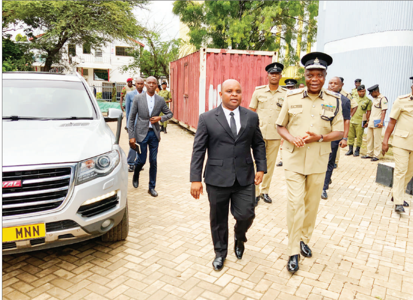
Home Affairs deputy minister Khamis Hamza Chilo (L) accompanied by Inspector General of Police Simon Sirro arrive to inspect construction of police headquarters in Dodoma yesterday. Photo: HoA
