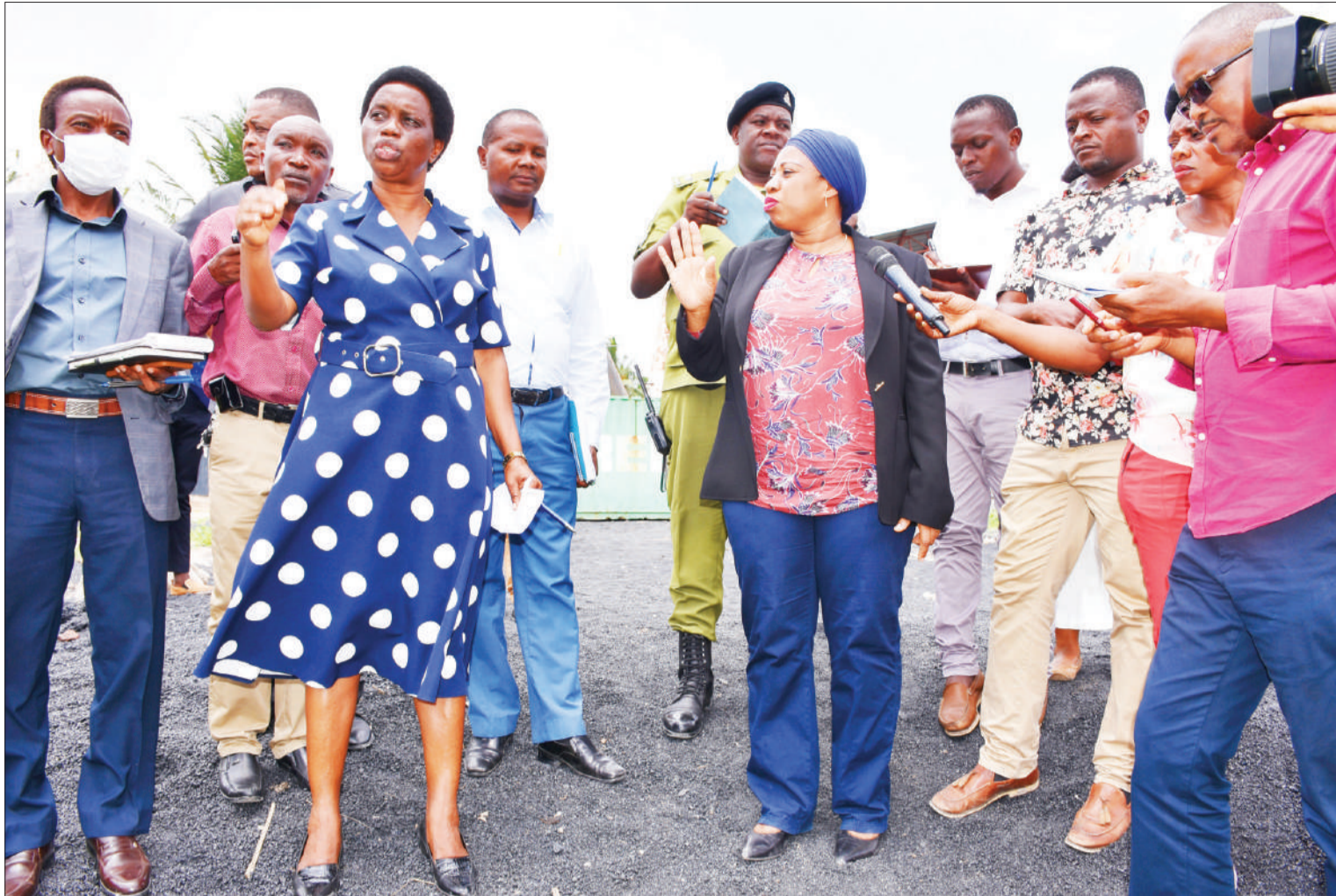
Vice President's Office (Union and Environment) minister of State Umyy Mwalimu (C) gets a briefing from Kibaha town council Director Jenipha Omolo on construction of a dump site on Tuesday. Photo: Guardian Correspondent
