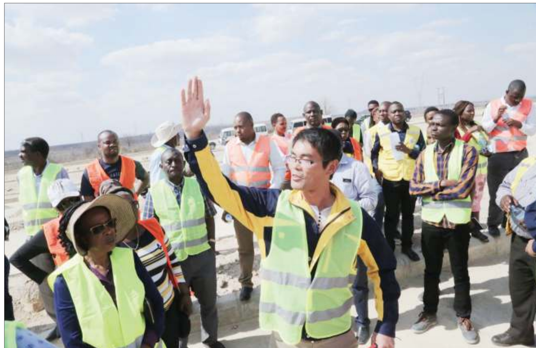
Xu Lei, a supervisor with Chinese construction firm Stecol Corporation, takes World Bank officials and President's Office (Regional Administration and Local Government) engineers around the site meant for development into a parking lot for heavy-duty trucks at Nala in Dodoma city yesterday. Sources said the lot will have capacity to accommodate 300 trucks at a time. Photo: Correspondent Ibrahim Joseph
