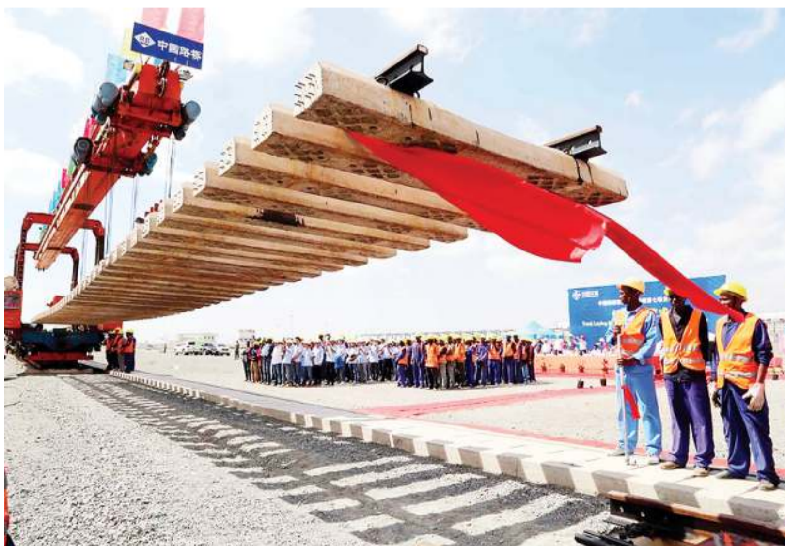
Standard gauge tracking laying in Kenya
