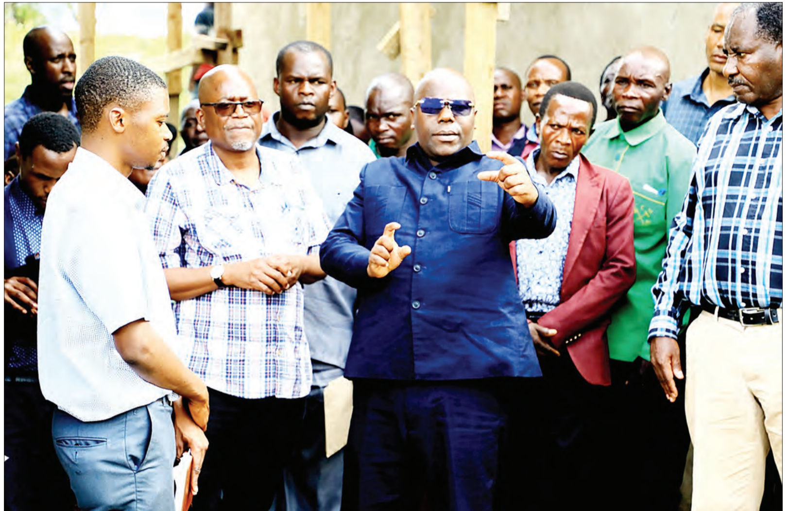
Mbeya Regional Commissioner Juma Homera gives orders to Busokelo Council engineer (not named) in Rungwe District on the construction of classrooms of Lupata secondary school. The school expects to enrol Form One students next year. Photo: Correspondent Nebart Msokwa
