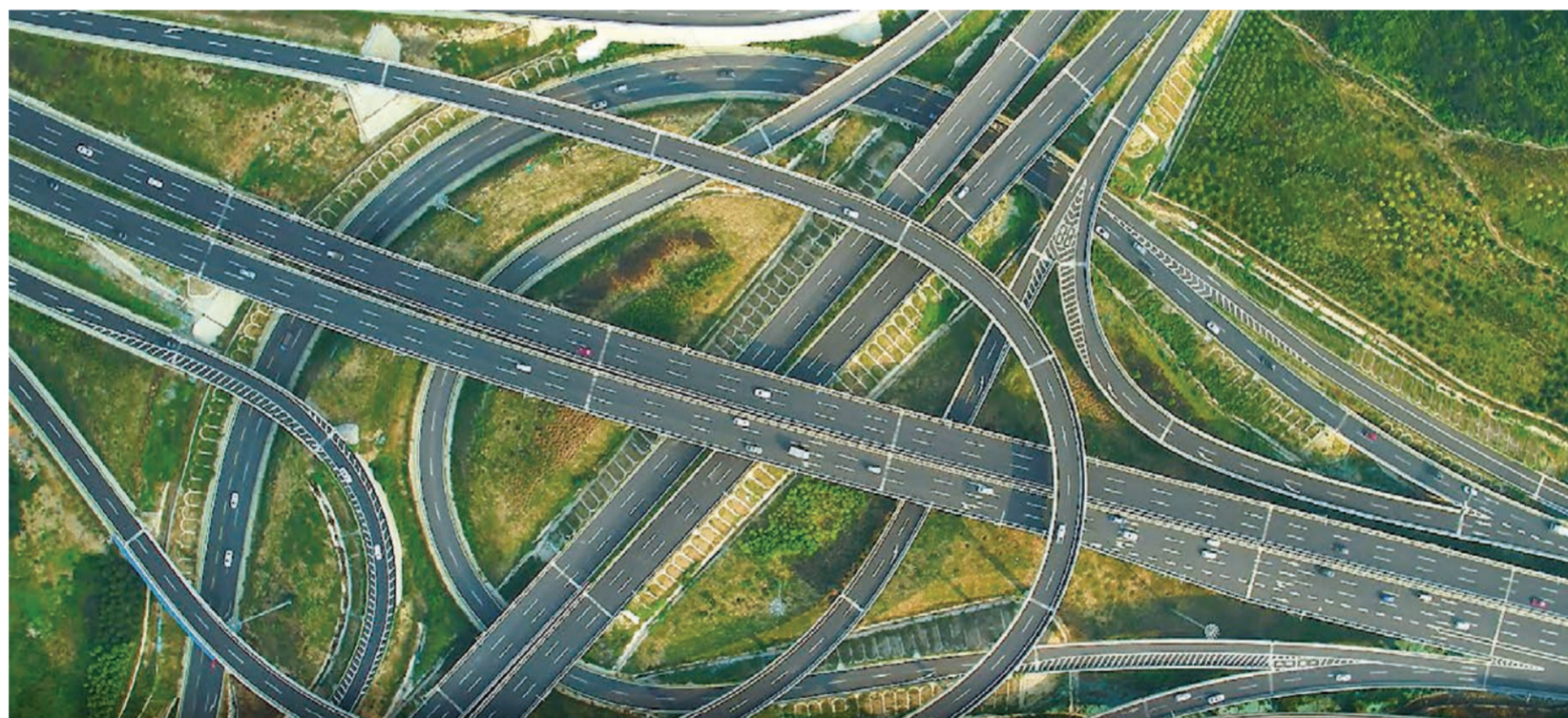
Photo shows a bird's-eye view of Beijing-Taipei expressway, a smart expressway that is expected to link Beijing and Taipei, southeast China's Taiwan, upon completion. Photo courtesy of Shandong Hi-Speed Group
