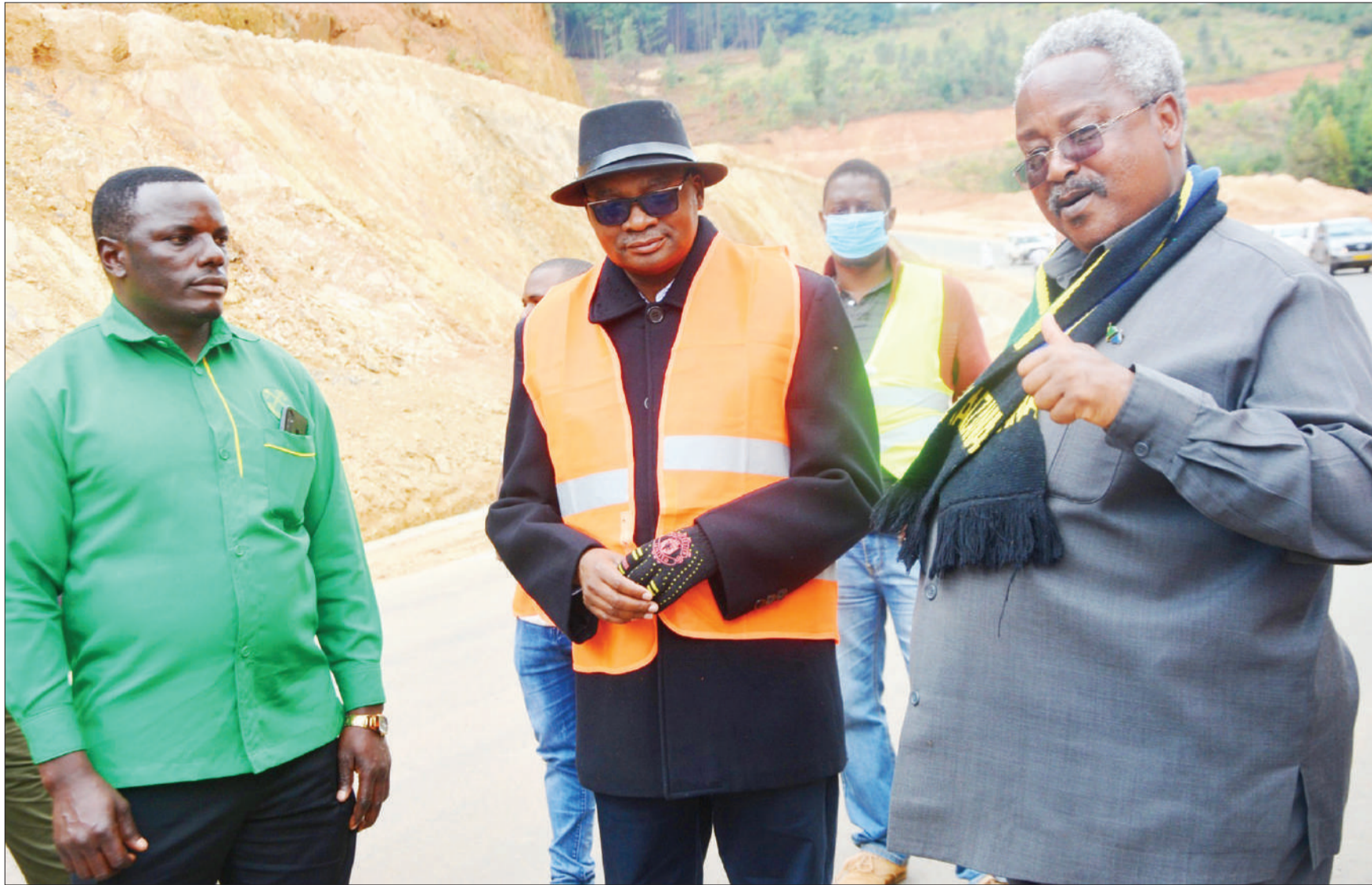
Njombe regional commissioner Christopher ole Sendeka (R) has a word with Works, Transport and Communications deputy minister Elias Kwandikwa (C), who was on inspection tour of the construction of the 107.4-km Njombe-Moronga-Makete road yesterday. Photo: Guardian Correspondent
