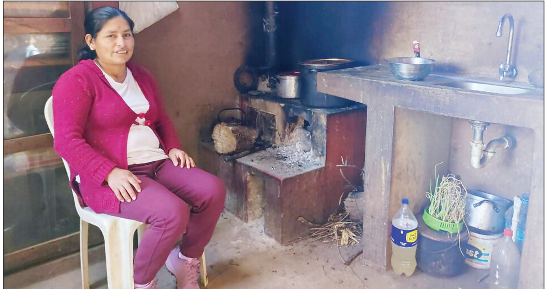
Martina Santa Cruz, a peasant farmer from the village of Saclo in the southern Peruvian Andes highlands department of Cuzco, is pleased with her remodeled kitchen where a skylight was created to let in sunlight and a chimney has been installed to extract smoke from the stove. CREDIT: Janet Nina/IPS
