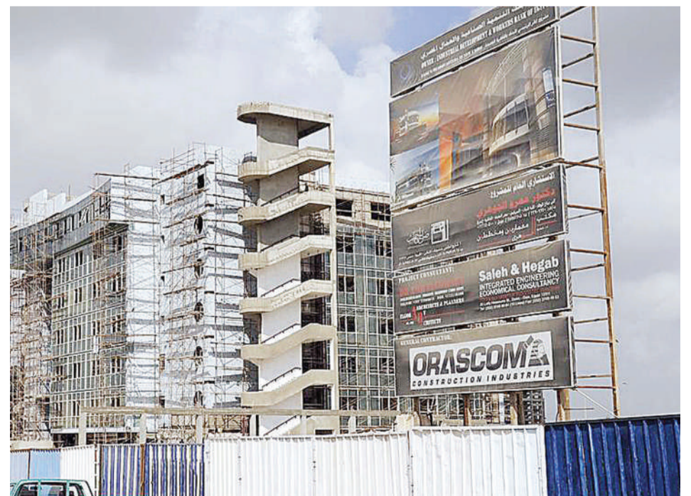
Egypt's Orascom Construction site in Cairo.
