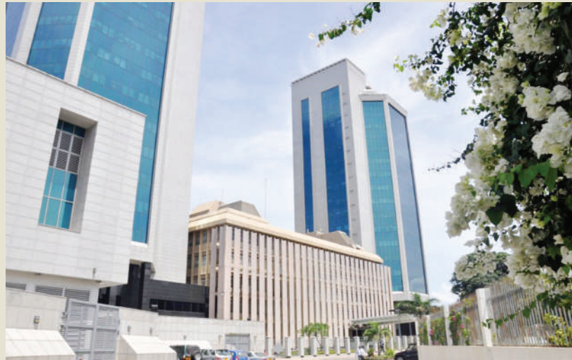
Bank of Tanzania headquarters in Dar es Salaam PHOTO/FILE
