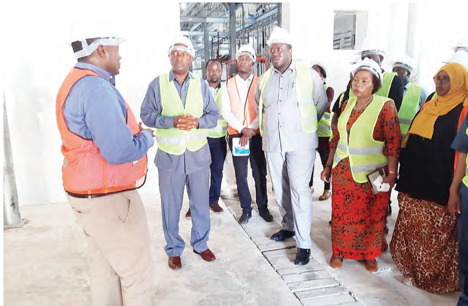
Tanchoice meat factory managing director Rashid Abdullah (L) briefs Coast regional commissioner Evarist Ndikilo (2nd-L) during a tour they made yesterday to a 1.1bn/- Dar es Salaam Water and Sanitation Authority (Dawasa) project meant to supply water to the factory. Others are Coast regional administrative secretary Theresia Mbandu (2nd-R) and Dawasa CEO Cyprian Luhemeja (3rd-L). Photo: Guardian Correspondent
