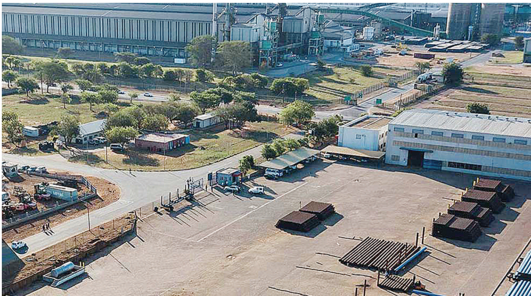
Beluluane Industrial Park in Mozambique.
