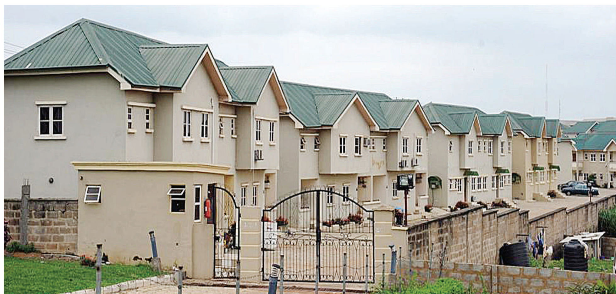
New residential apartments in Lagos.
