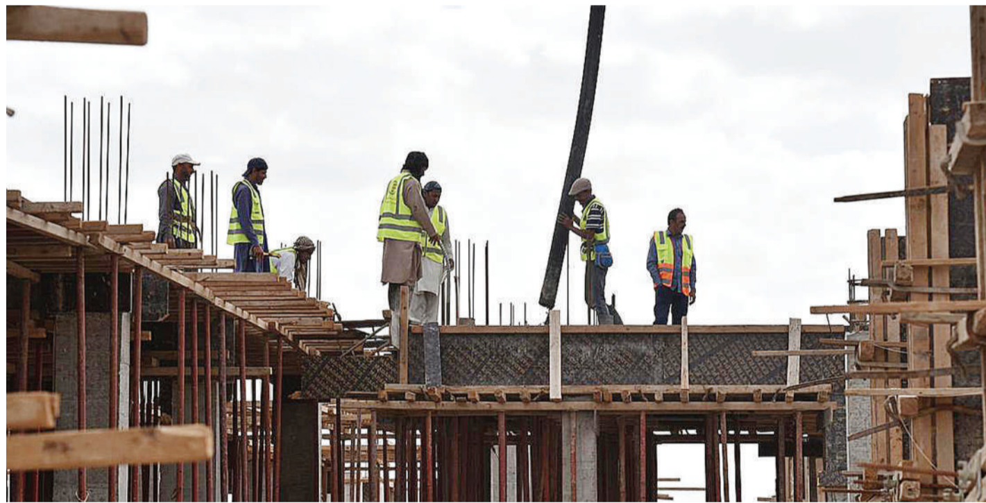
Work in progress at a construction site in Riyadh
