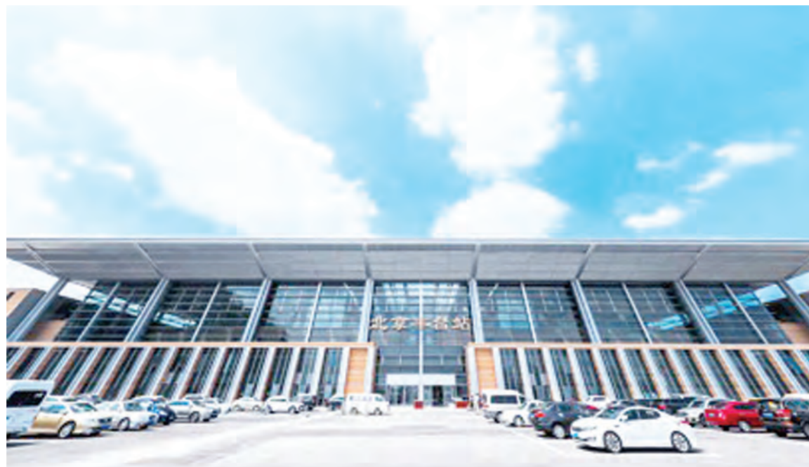
Photo taken on June 14 shows the exterior of the Beijing Fengtai Railway Station.
