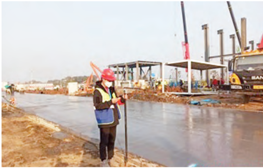
An engineer is surveying at the construction site of the makeshift hospital Leishenshan in Wuhan with a BDS-based device.
