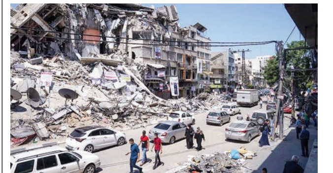
Motorists and pedestrians move past a building destroyed by an air-strike prior to a cease-fire that halted the 11-day war between Gaza's Hamas rulers and Israel, May 25, 2021, in Gaza City, the Gaza Strip. (File photo)
