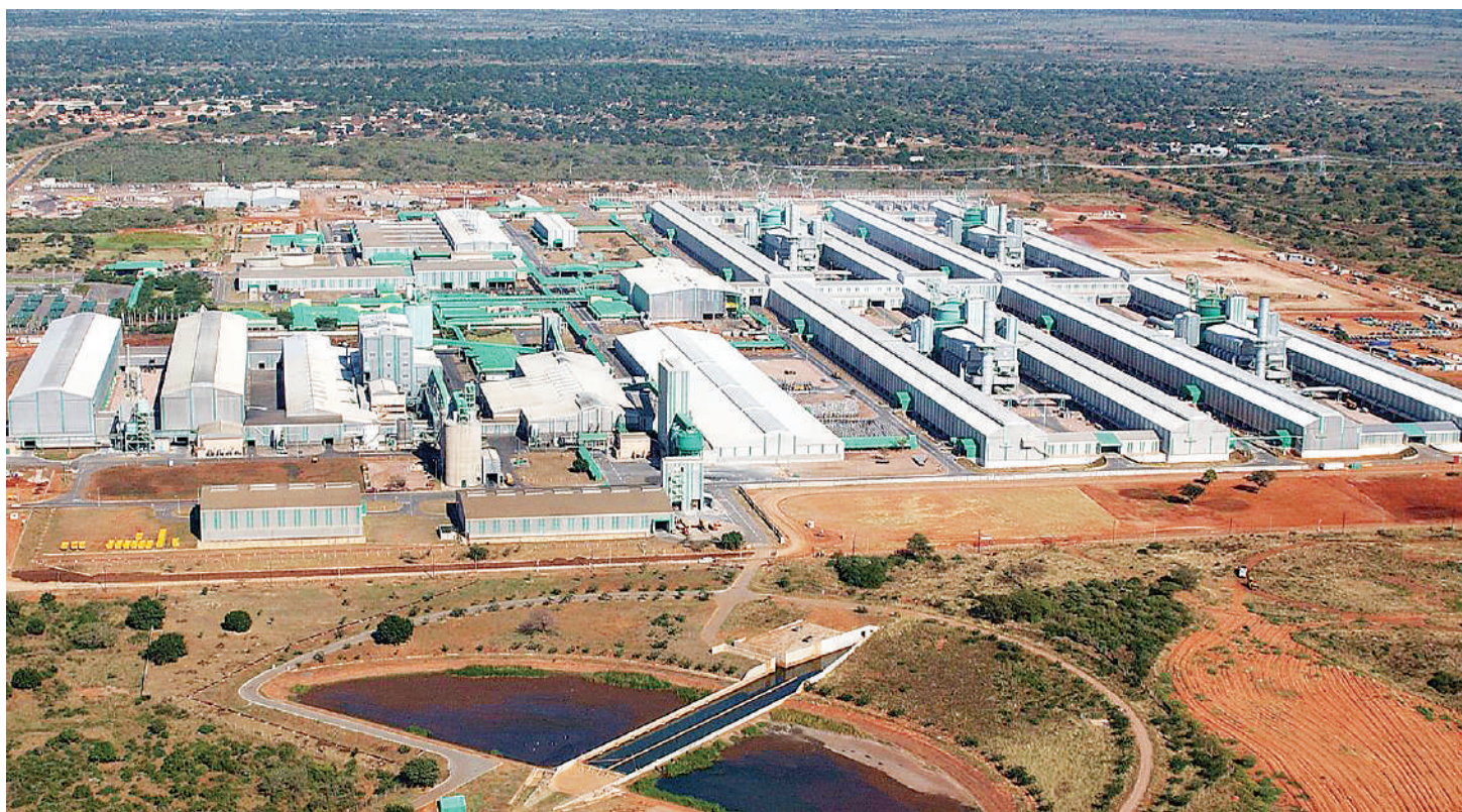
Beluluane Industrial Park in Maputo where Raxio plans to locate its data centre.
