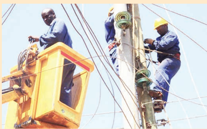
Kenya Power workers connecting new homes in rural Naivasha.
