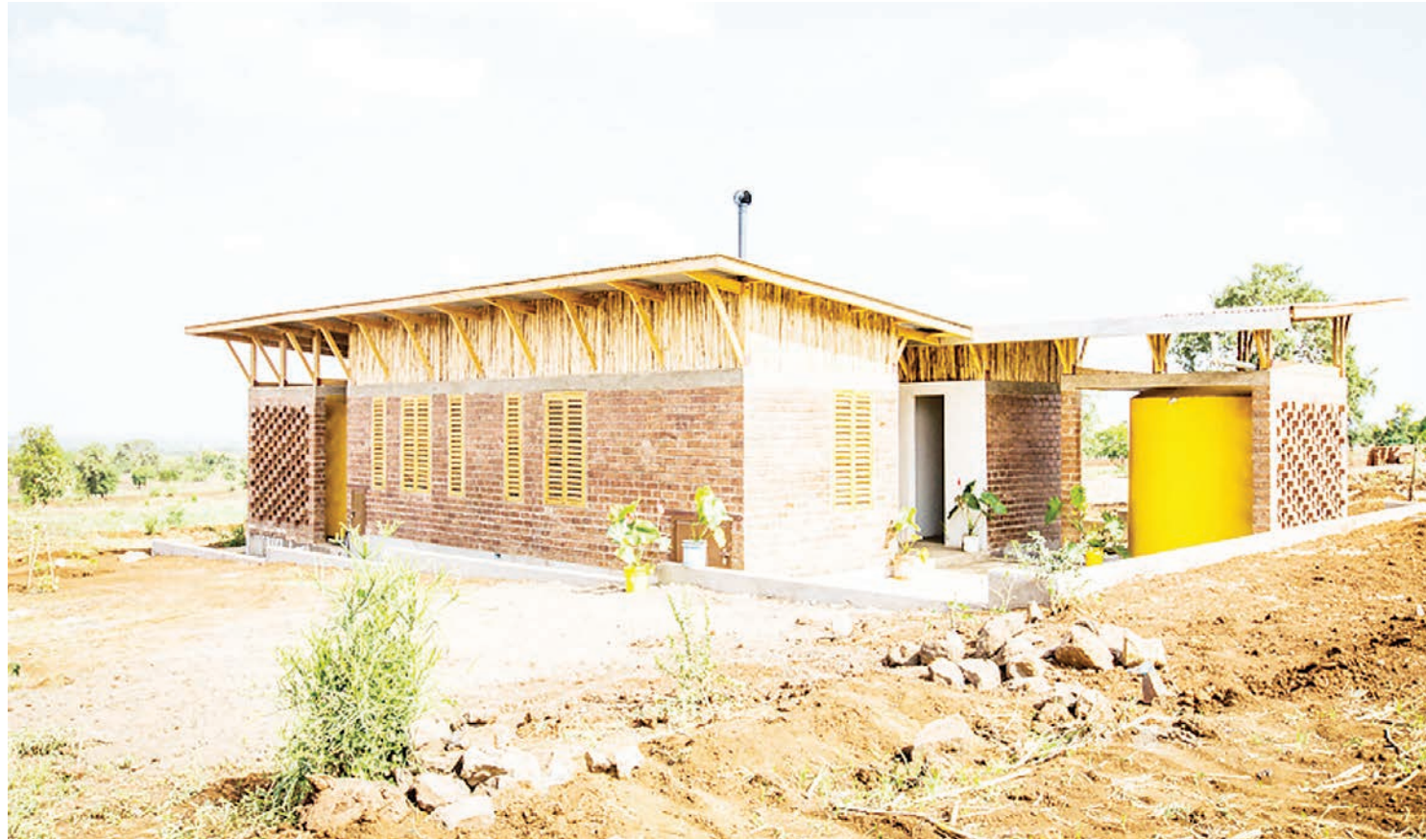
A bamboo built structure in rural Tanzania.
