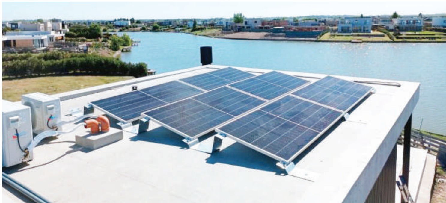
Aerial view of the 5000 square meter roof full of solar panels, in one of the pavilions of La Rural, the busiest fair and exhibition center in Buenos Aires. It is the largest private solar park in the capital of Argentina and required an investment of almost one million dollars.
