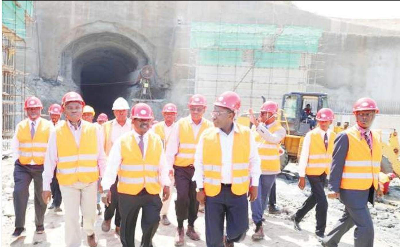
Energy minister Dr. Medard Kalemari (2nd L), Burundi Energy and Mining minister Come Manirakiza (L) and Rwanda Infrastructure Minister Claver Gatete (3rd R) after their tour at the proposed construction of 80 MW electric plant at Rusumo within the border of Rwanda and Tanzania. Photo: Correspondent Teresia Mhagama
