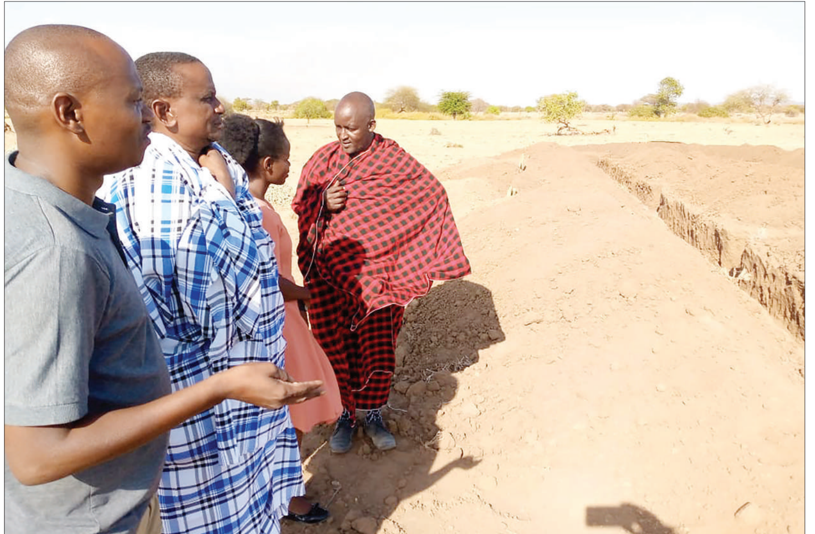
Billionaire tanzanite miner Saniniu Laizer (2nd-L) of Mirerani in Simanjiro District makes an on-site inspection on Wednesday of preparations for the government-funded construction of a Saniniu Laizer Primary School dormitory in Naisinyai ward. Photo: Correspondent Gift Thadey
