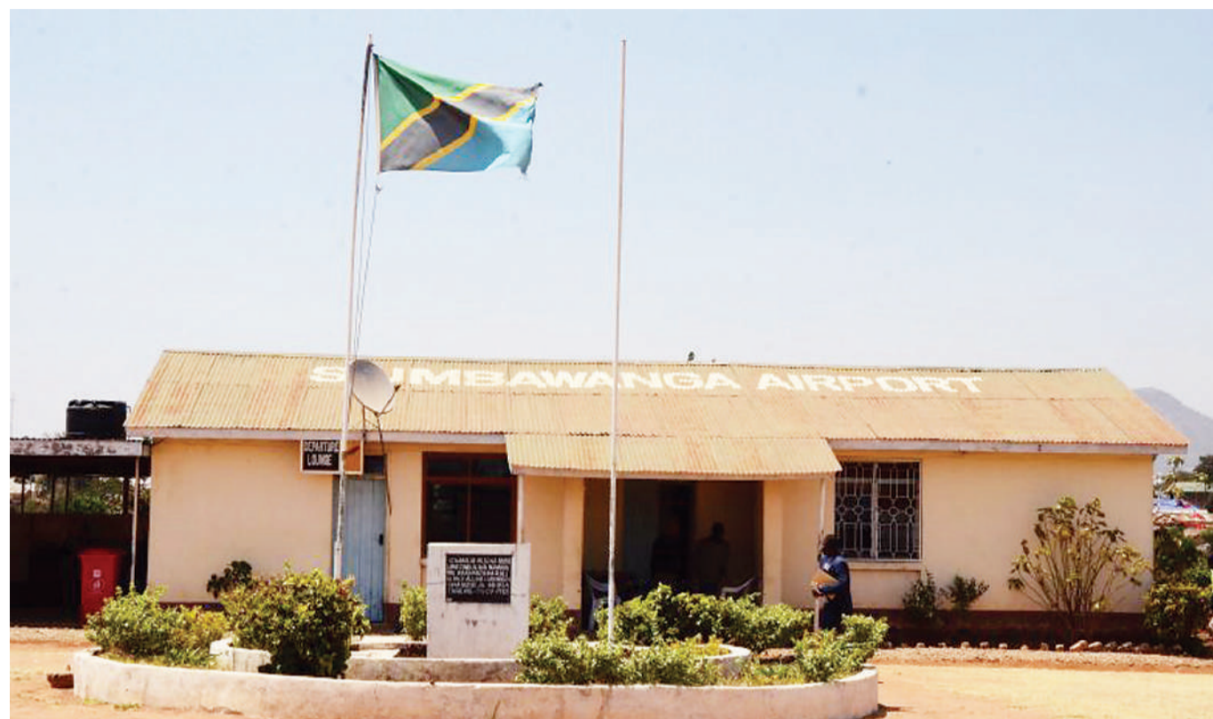
Sumbawanga Airport office building
