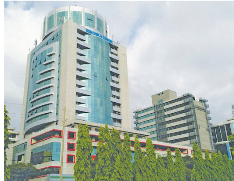
A side view of the TFC Tower in Dar es Salaam.
