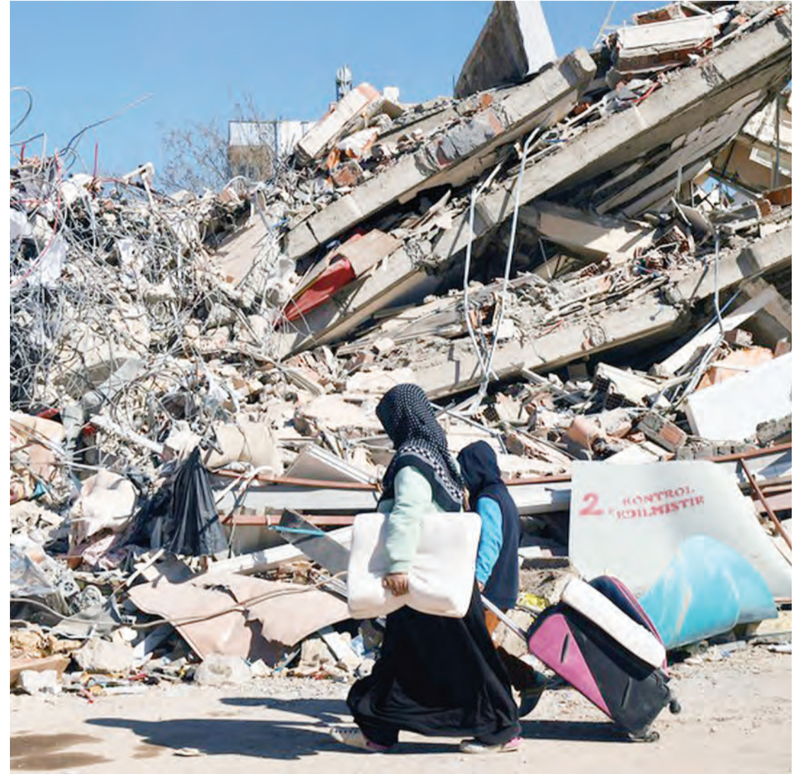
People walk past a collapsed building in Adiyaman, Türkiye, Feb. 18, 2023. (Photo by Mustafa Kaya/Xinhua)
