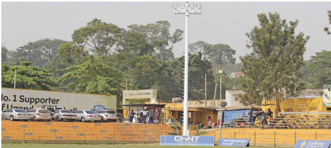
The new floodlights at the MTN Omondi Stadium in Lugogo.
