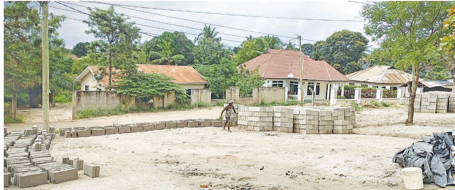
John Nkindikwa (36) laying concrete blocks at Gewe Vibrated blocks in Matosa suburb of Dar es Salaam. Photo: Francis Kajubi.
