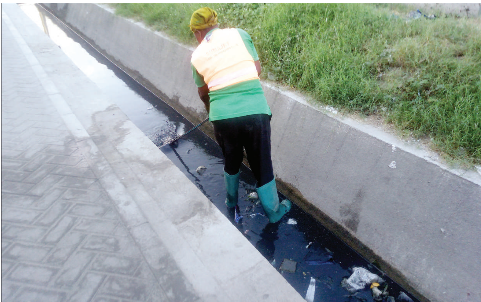
Clearing of a rainwater trench beside a Mwenge section of Dar es Salaam's Ali Hassan Mwinyi Road gets slowly under way yesterday. Photo: Correspondent Sabato Kasika
