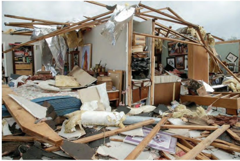
The damaged remains of the Walnut Ridge neighborhood is seen on Saturday in Little Rock, Arkansas. (PHOTO / AFP)
