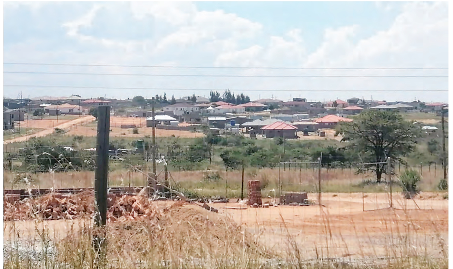
Upmarket houses built by members of the urban elite in Limpopo's Capricorn West district. (Photo Supplied)
