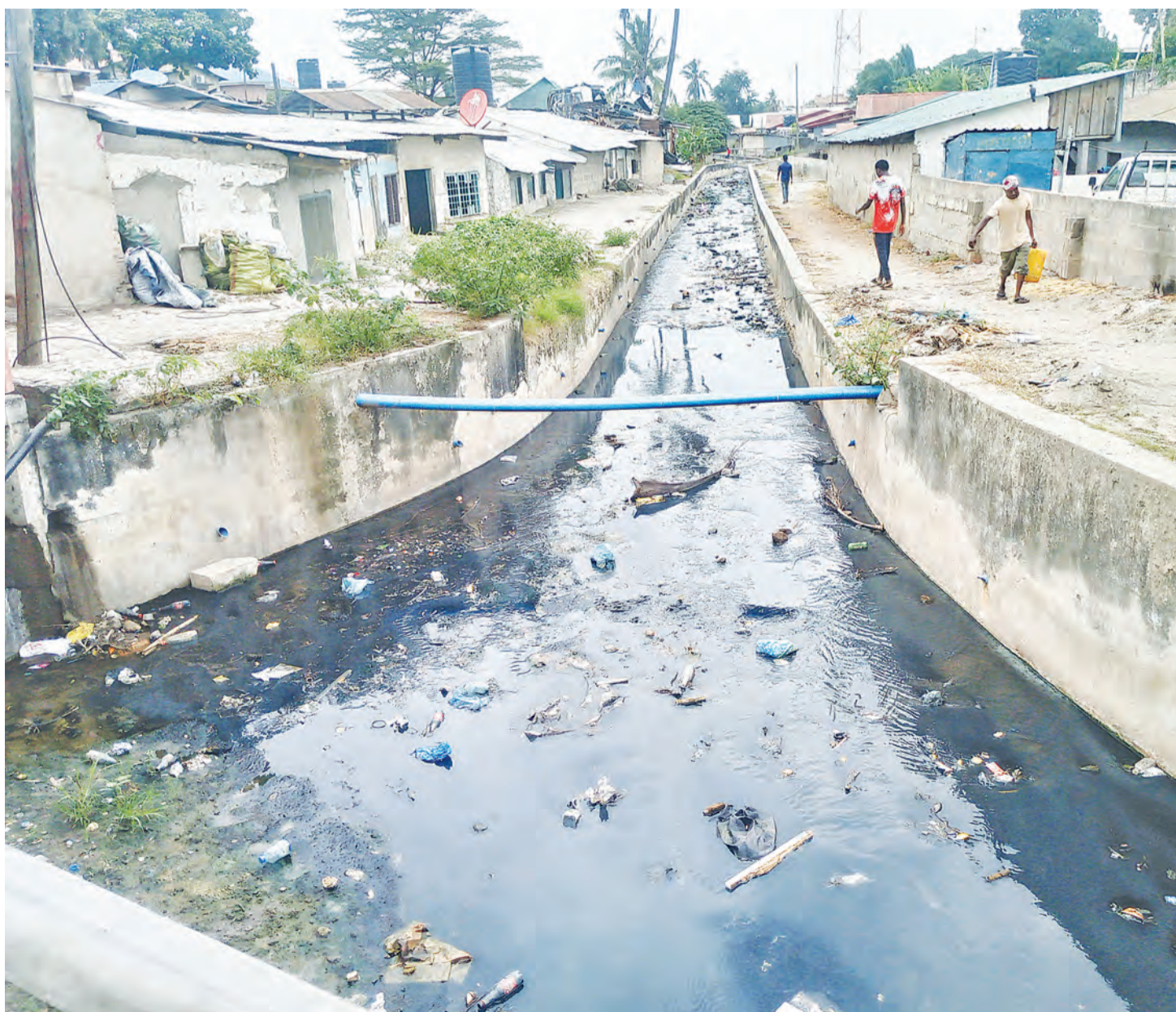
This trench, found deep inside the Uzuri Kilimani segment of Dar es Salaam city's densely populated Manzese suburb, has for long turned into a virtual "river" of sewage mainly discharged from toilets that is seriously endangering public health. Correspondent Sabato Kasika captured the scene yesterday
