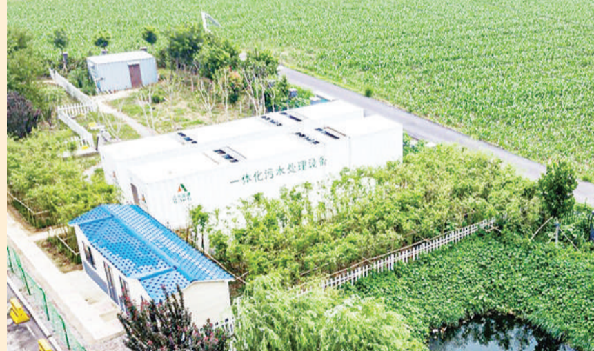
Photo shows the wastewater treatment facility of the Jinan East carbon-zero service station. (Photo provided by Shandong Hi-Speed Company Limited)
