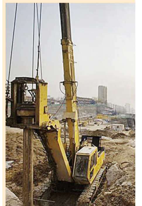
A construction site in Johannesburg.
