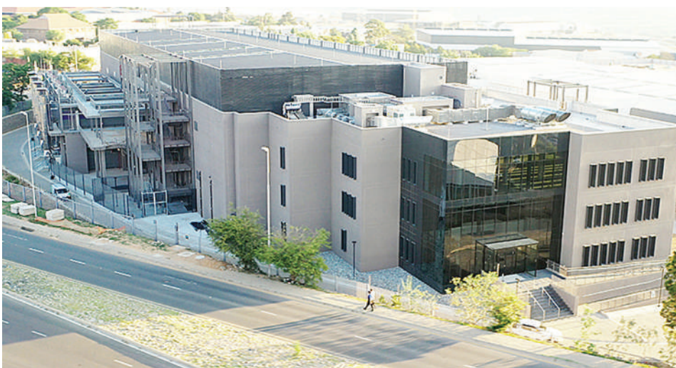
The recently completed 10MW JHB1 Africa Data Centres facility in Midrand.
