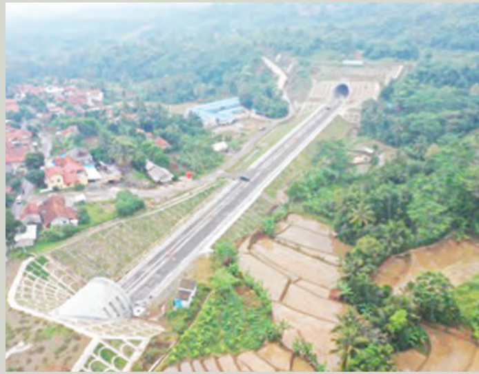
Tunnel No. 6, the longest tunnel of the Jakarta-Bandung High-Speed Railway is completed, Feb. 18, 2022. (Photo by China Railway No. 3 Engineering Group Co., Ltd.)
