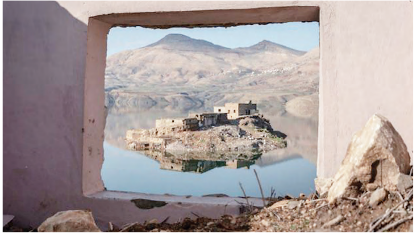
Water scarcity in the Middle East is impacting on lives and causing diplomatic tensions in between countries. The Turkish dam project, which includes the large Ataturk and Ilisu dams, has reduced water flow to the Tigris River's natural channel impacting Syria and Iraq. Pictured here is Koctepe - a village covered by water in the Ilisu dam project. Credit: Mustafa Bilge Satkin/Climate Visuals Countdown
