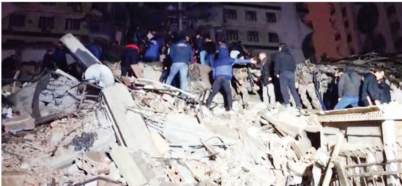
In this video grab from AFP TV taken yesterday, rescuers search for victims of a major earthquake that hit Diyarbakir, in southeastern Türkiye, leveling buildings across several cities and causing damages in neighboring Syria. (PHOTO / AFP / AFP)
