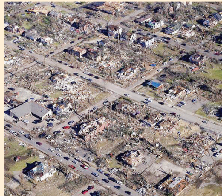
In this aerial photo, destruction in downtown Mayfield, Kentucky is seen on Sunday in the aftermath of tornadoes that tore through the region. AP
