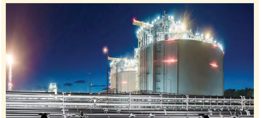
A liquefied natural gas storage. File Photo
