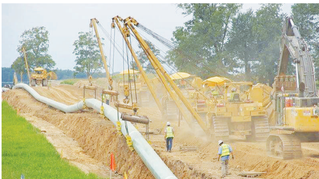
Ongoing construction works of the East Africa Crude Oil Pipeline
