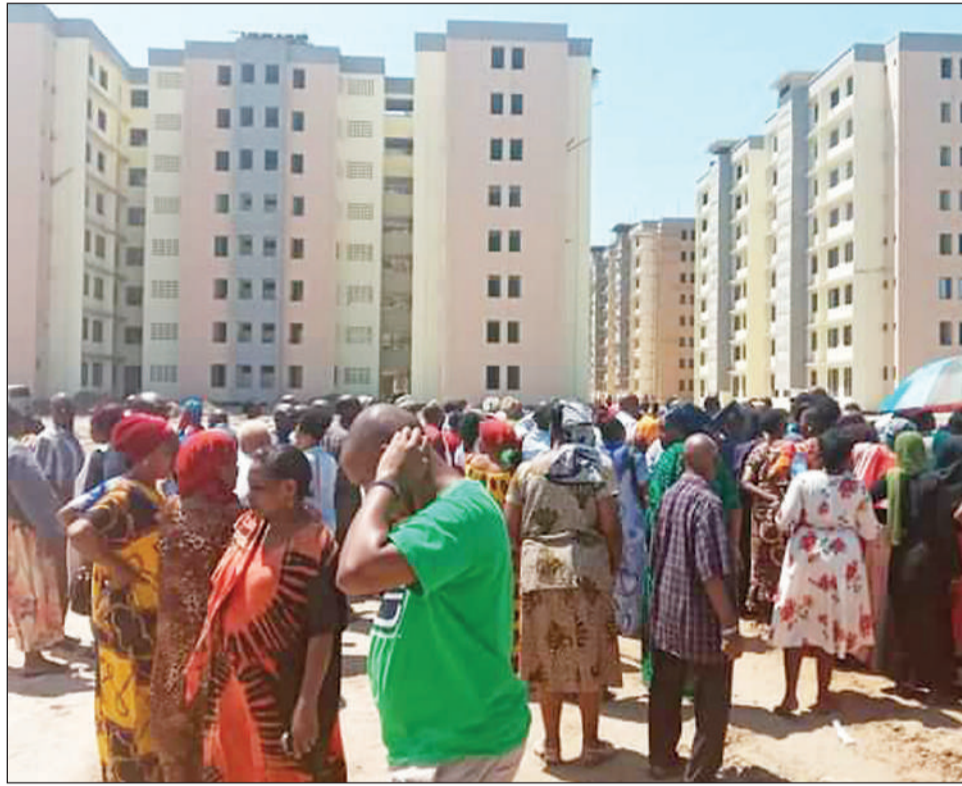
Residents of Magomeni Quarters verifying their documents at the site of their prospective new apartments in Dar es Salaam earlier this week. Photo: Guardian Correspondent.
