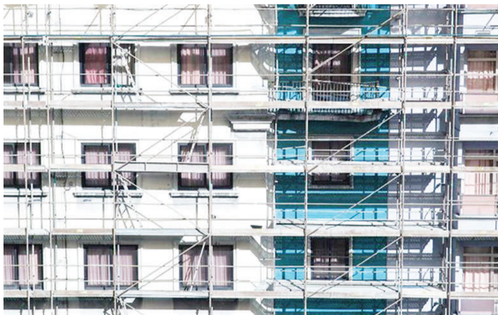
A residential apartment under renovation in Nairobi.
