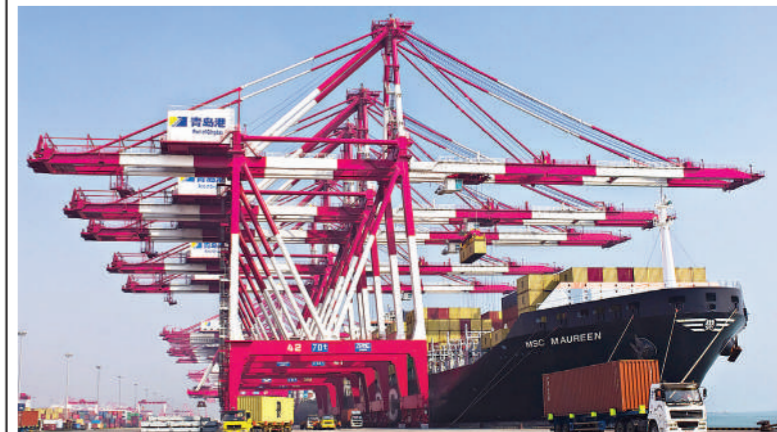
Qianwan Container Terminal in Qingdao, China
