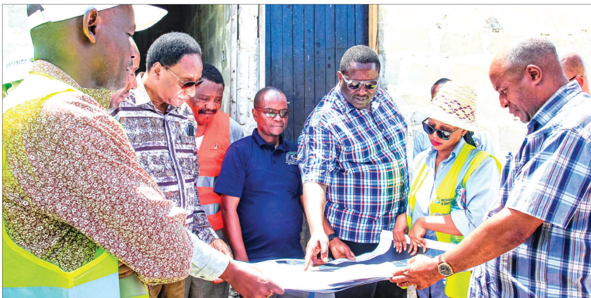
Dar es Salaam Water and Sanitation Authority (Dawasa) CEO Cyprian Luhemeja (3rd-R) briefs the board chairman, former Chief of Defence Forces Davis Mwanunyangye (2nd-L, foreground), on the Makongo-Bagamoyo water project. This was during Monday's inspection tour by Dawasa board members. Photo: Correspondent Joseph Mwendapole
