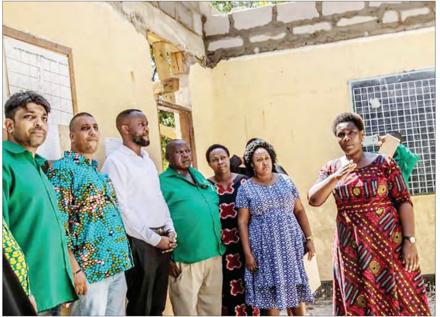
Kivukoni Ward Councillor Sharik Choughule (2nd L) and his delegation listen to Bunge primary school head teacher Leonida Mulekuzi (R) during their visit to inspect the ongoing renovation of the school in Dar es Salaam yesterday. The funding of the renovation was provided by the City Council. Third (L) is the councillor and chairman of social services Robert Manangwa and CCM's Ward political committee members. Photo: Guardian Correspondent
