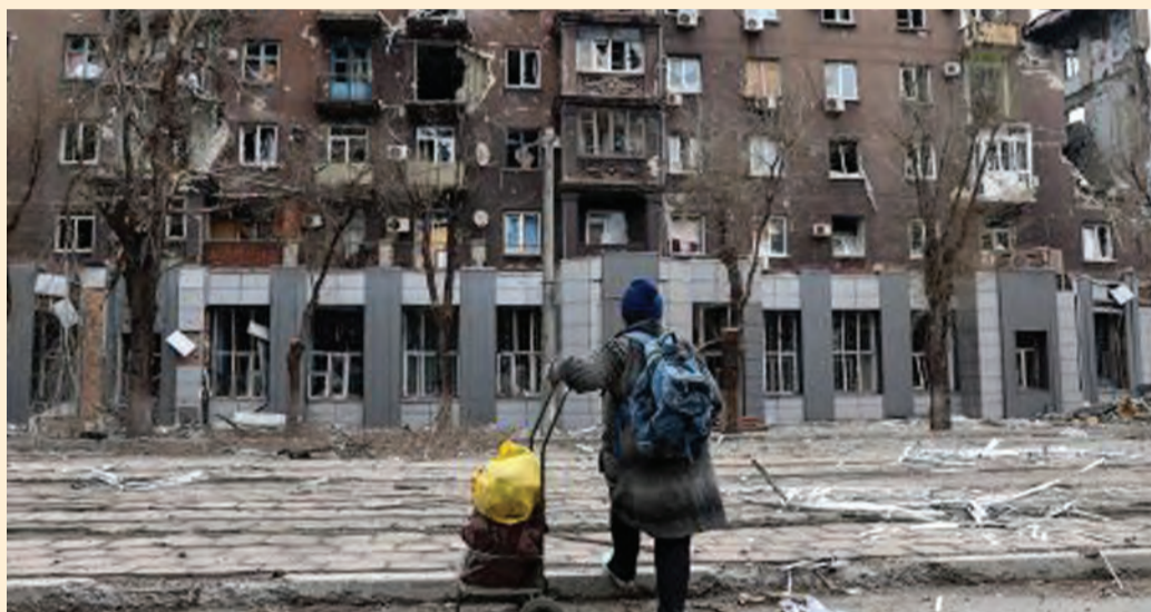
A local resident looks at a damaged apartment building near the Illich metallurgical plant in Mariupol on April 16, 2022. File photo
