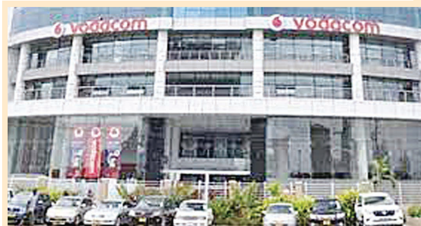
Vodacom Tanzania Plc's head office in Dar es Salaam.
